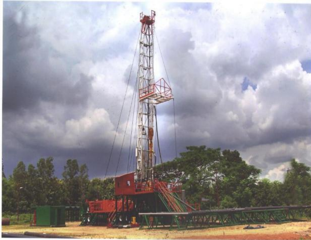
Drilling Rig in operation at Moonidih
