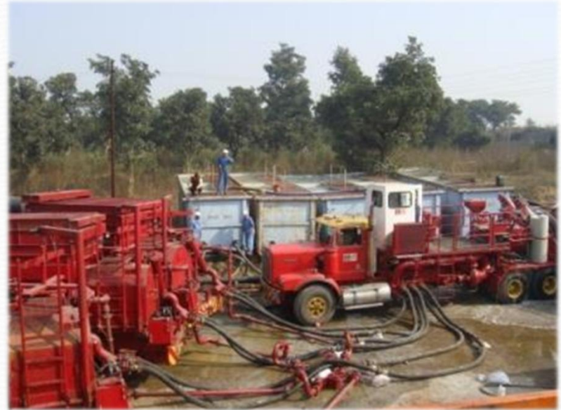
Hydro-fracturing unit at CBM Well
